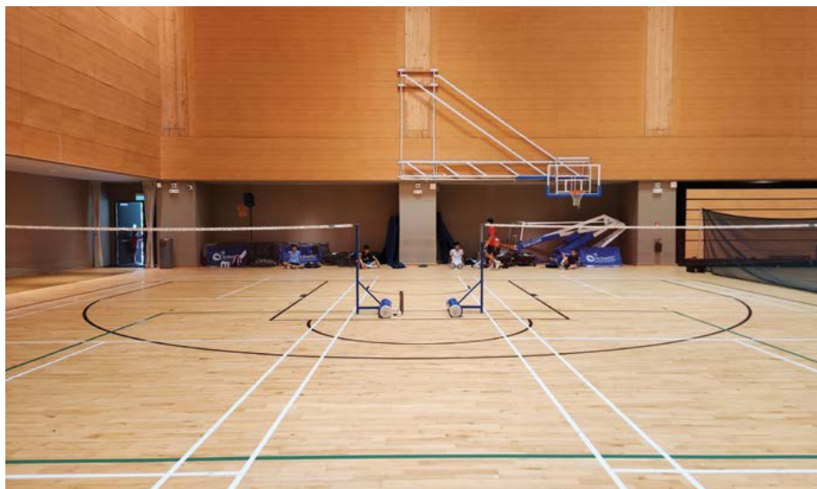
Sports hall designed for multiple sports, finished with American maple flooring with CLT walls
